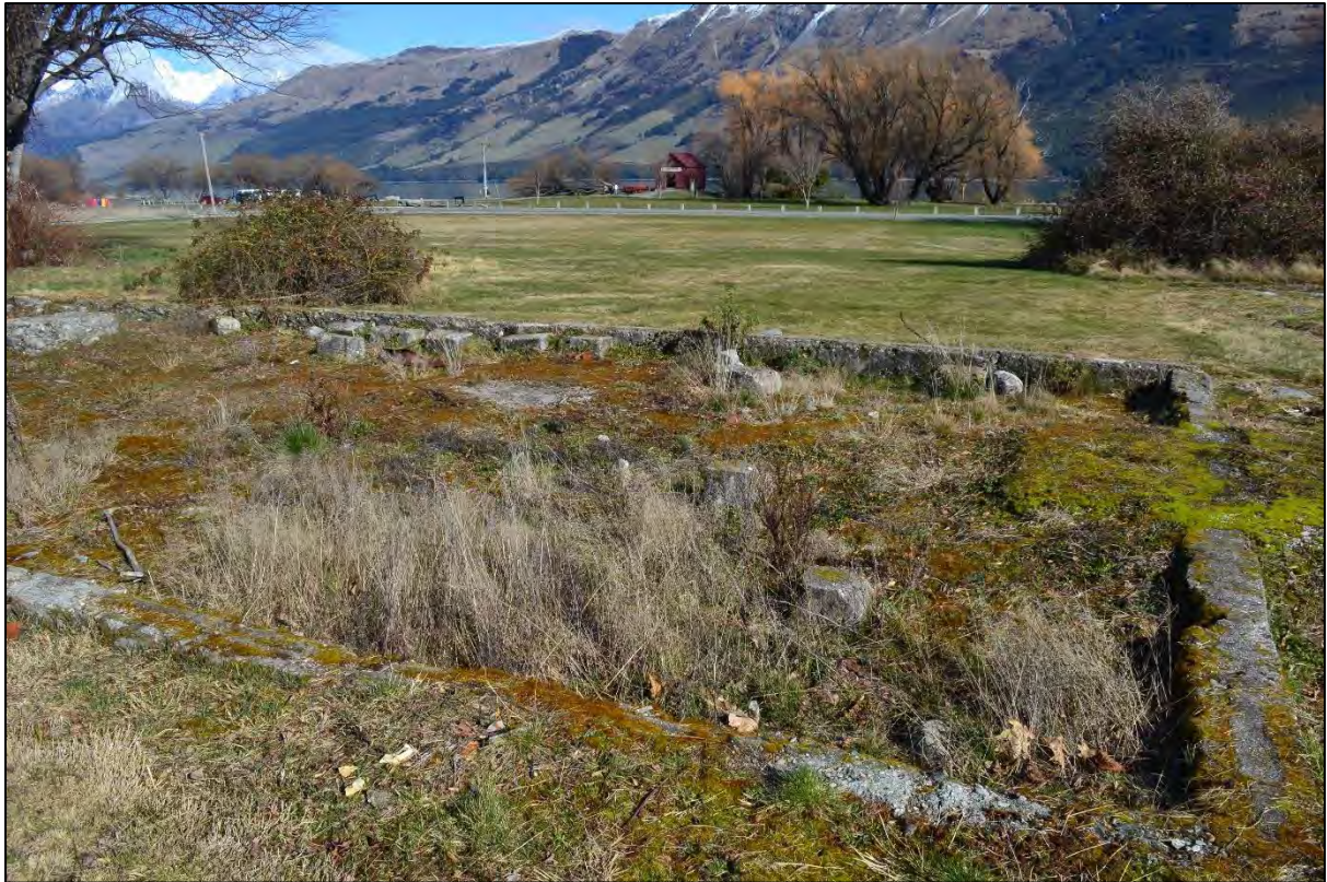
Figure 24. Detail of concrete ring foundation with internal concrete piles and foundation of large chimney on northern edge.
