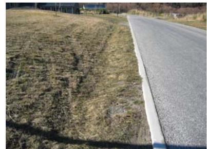
Adopt grass drainage swale and flush concrete edge to seal. Instead place concrete beneath seal edge.
