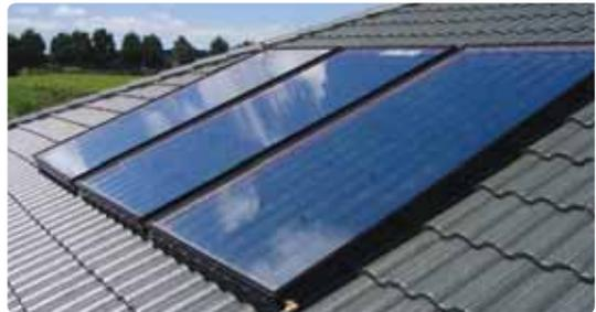
Frame-mounted flat plate collector panels.
