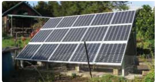
This photovoltaic array uses an inclined frame mounted on the ground.
