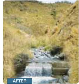
Simulation of the impact a micro (2-5kW) hydro scheme could have, looking upstream. A small weir is constructed to divert a portion of the stream into a penstock.
