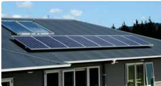
A PV array installed directly onto the roof.
