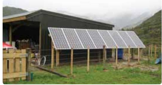
An example of a frame-mounted PV array on the ground.
