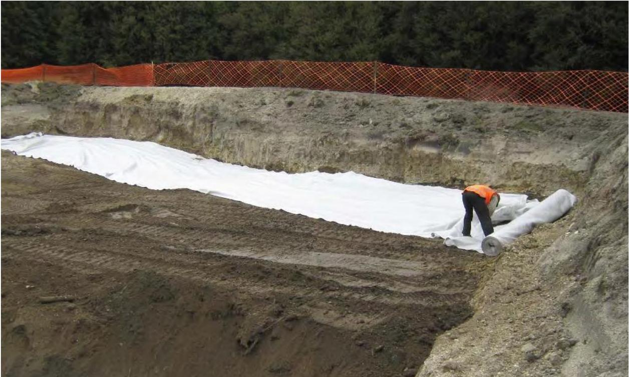
Mixed soils depository and placement of geotextile fabric as visual indicator
