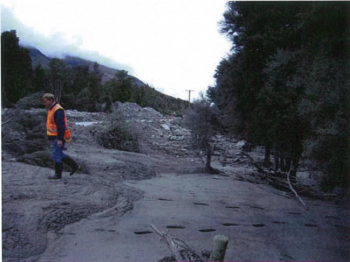
**Figure 27: Debris on true right of Pipson Creek at SH6, showing depth of flows during 2006 event.**
