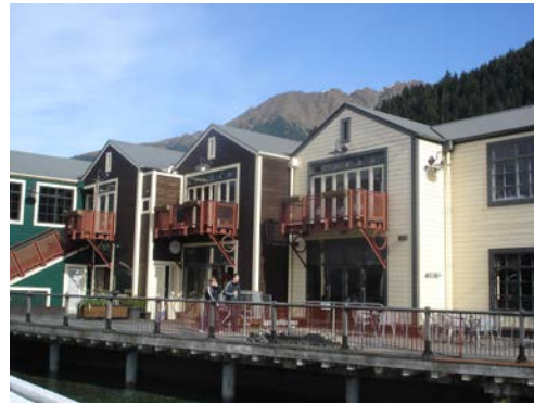
Steamer Wharf, 88 Beach Street
