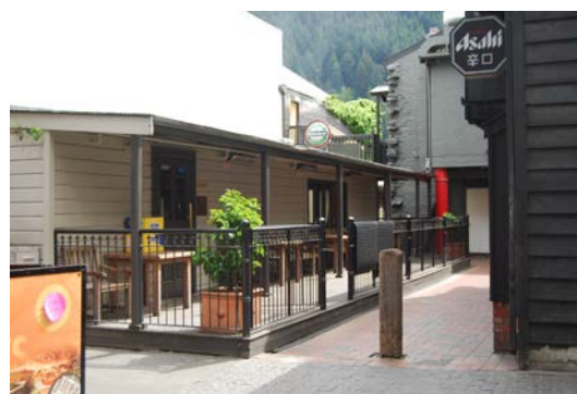
Pedestrian Arcade from Searle Lane to Mall
