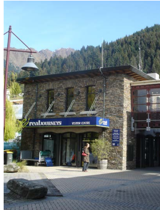
Steamer Wharf, 88 Beach Street
