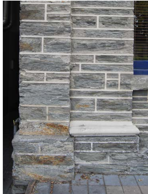
Council Chambers, 50 Stanley Street (tuck-pointing)
