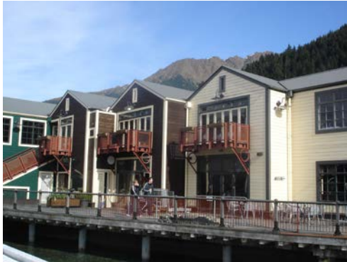
Steamer Wharf, 88 Beach Street
