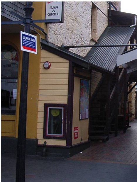
19, Ballarat St (painted weatherboards)
