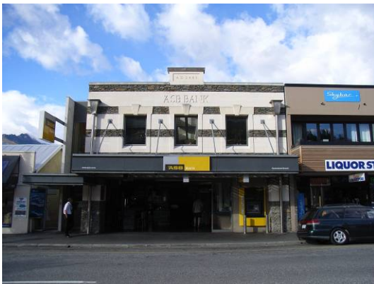
ASB Building, 24 Camp Street
