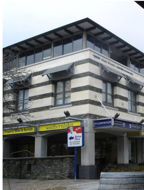
Ward Wilson Building, 10 Athol Street
