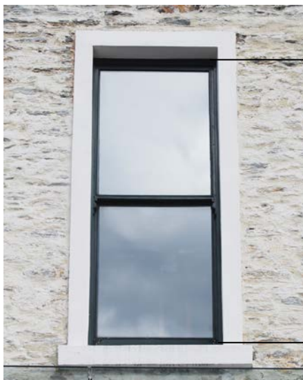
Mountaineer, 28 Rees St
