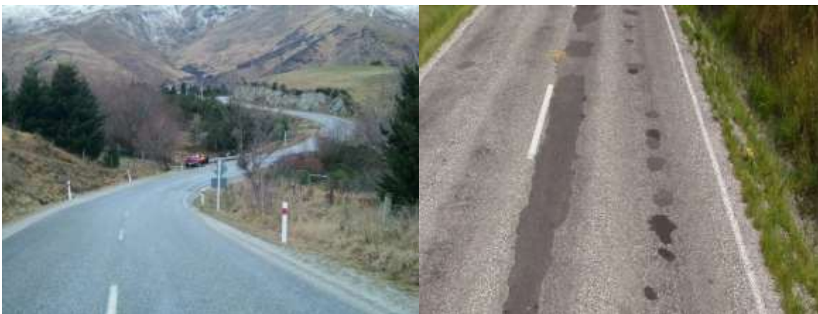
Photos of Royal Burn section and typical extent of pavement repairs
