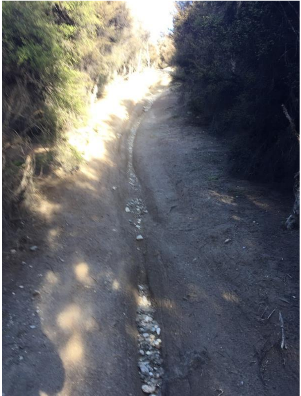
Photograph 9 – Photograph of erosion of bike track within gully below Lot 20. Track has been progressively widened by bikers avoiding rutted section.
