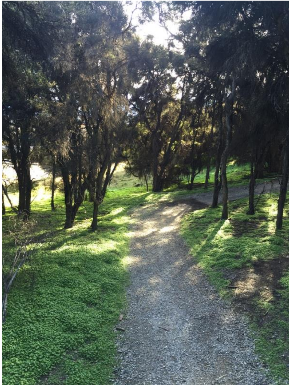
Photograph 1 – Example of track formation in Stage 3b of Peninsula Bay. Track formation is 1.5m. Removal of kanuka was keep to a minimum whilst still maintaining a canopy above the track by selective pruning of branches.
