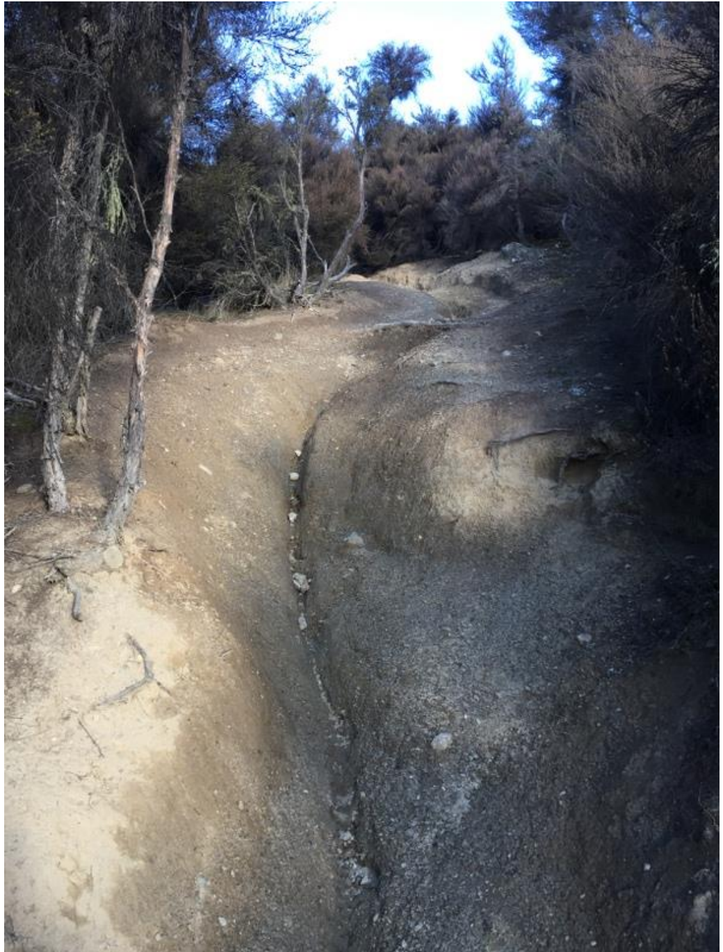
Photograph 10 – Photograph of erosion of bike track within gully below Lot 20. Track has been progressively widened by bikers avoiding rutted section. Track has 0.5m to 1m vertical drops.
