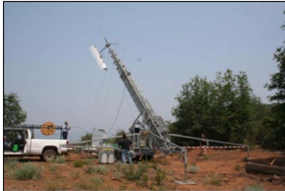
Figure 4: Temporary cellphone tower being erected in California to assist fire fighting
