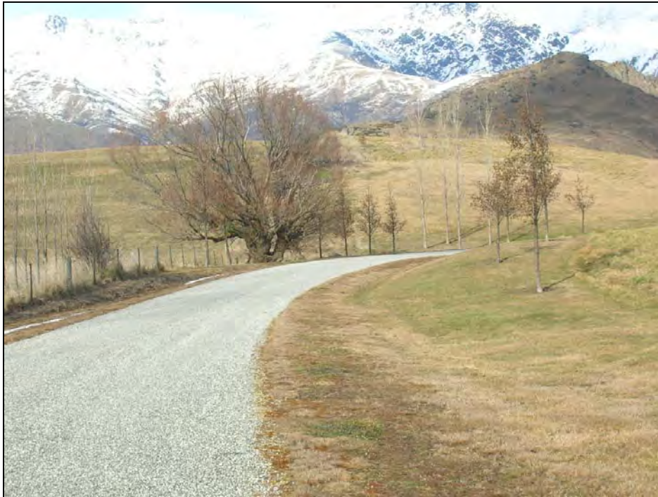
Photo 2: Roadside grass swales for stormwater
