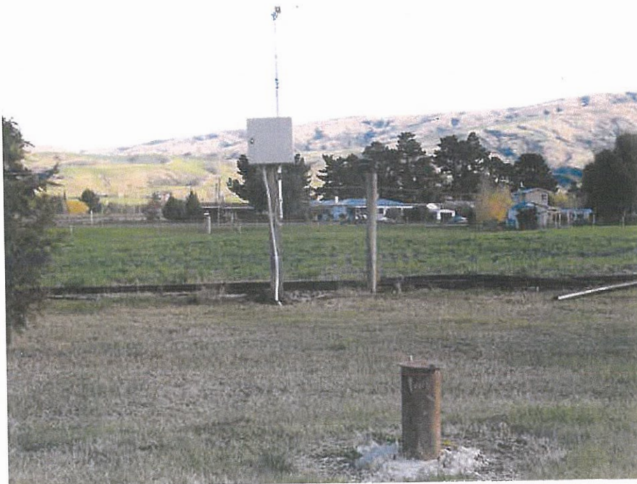
Figure 4: Example of finished bore and telemetry system.
