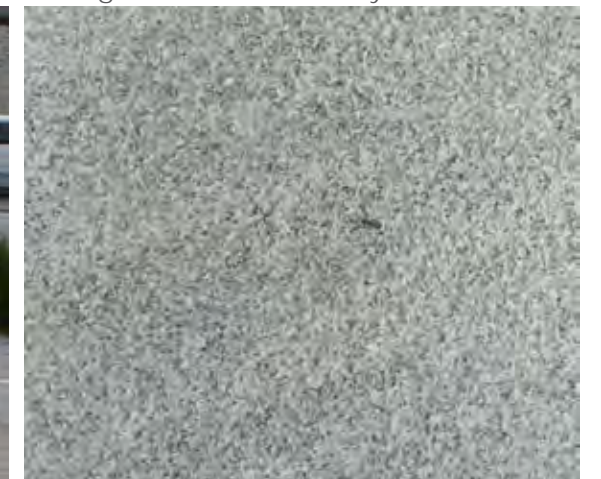
Exposed aggregate concrete pathways
