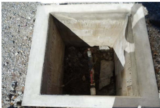
Borehead within concrete chamber. Borehead itself not sealed.
