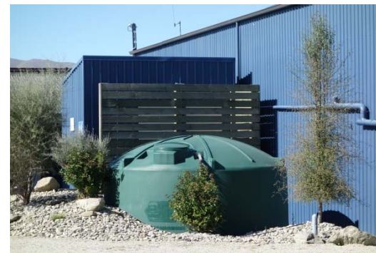
Plastic storage tanks like this one are located on each property for storage & firefighting.
