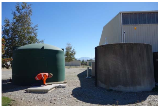
Borehead under steel lid, plastic firefighting storage tank & concrete storage tank (reservoir)
