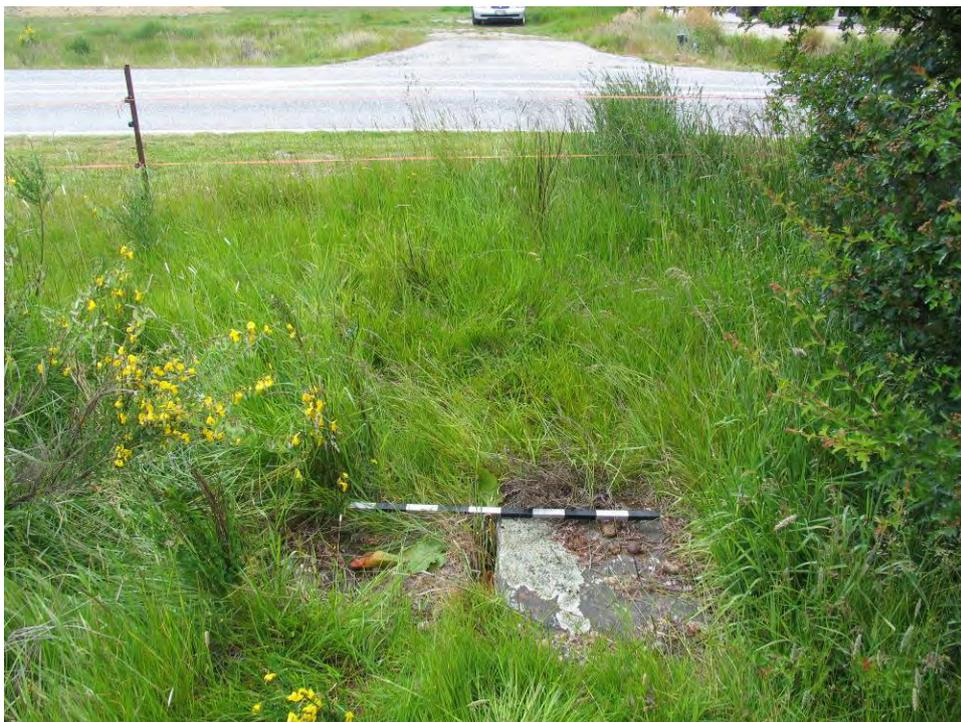
**Figure 12.** Schist crossing over culvert beside main road.
