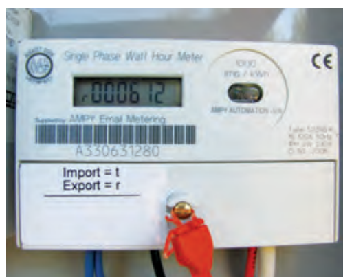
Figure 15. A typical two-way meter Photo credit: Contact Energy
