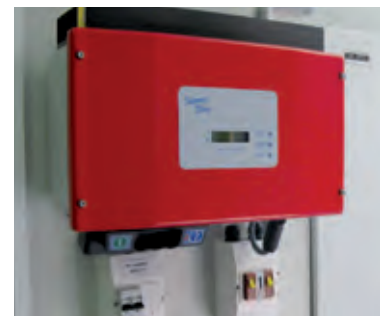
Figure 61. A Sunny-Boy inverter installation Photo credit: SolarQuip Ltd
