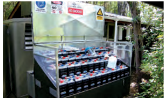
Figure 56. A battery bank in a SAPS Photo credit: Genkit Nelson Ltd
