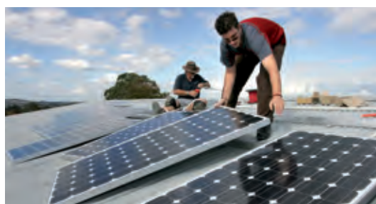
Figure 24. PV modules being installed on a roof Photo credit: Genesis Energy Schoolgen
