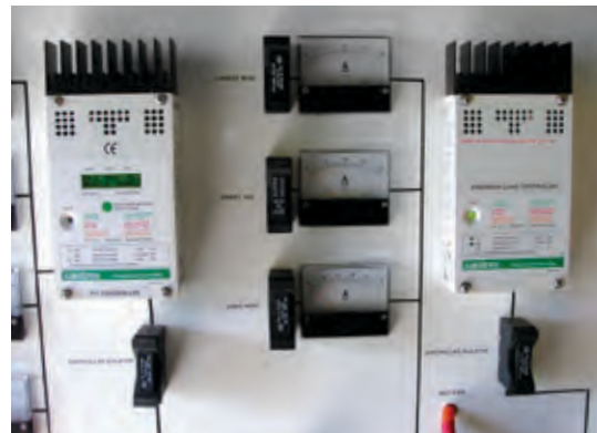
Figure 60. Controllers used on a PV-based system Photo credit: EcolInnovation
