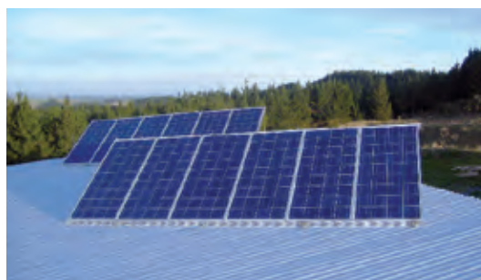
Figure 20. PV arrays installed in a SAPS Photo credit: Ecolnnovation
