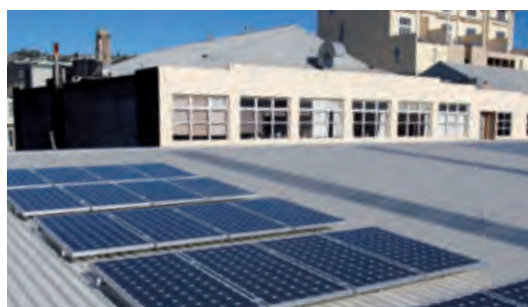
Figure 3. Part of the 10.5kW PV array installed on a Wellington supermarket. Photo credit: Joseph Mayhew
