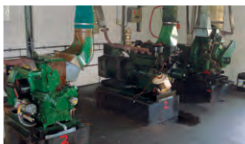
Figure 11. Diesel generators are commonly used with SAPS. Photo credit: Department of Conservation
