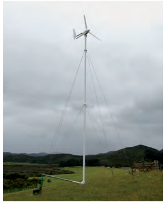
Figure 48. Pole-mounted micro wind turbine with tilting mechanism Photo credit: Gusto Energy Ltd
