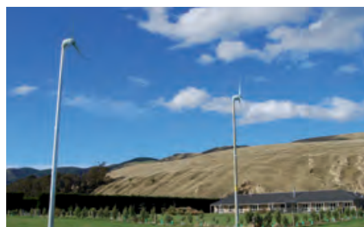
Figure 38. Two micro wind turbines in a grid-connected system near Christchurch Photo credit: Joseph Mayhew
