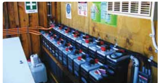
Battery bank on a SAPS. Photo: Genkit Nelson Ltd.
