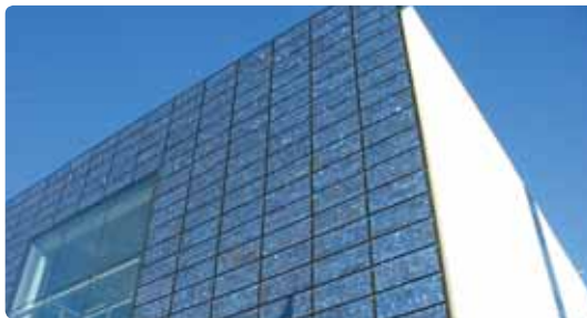
The façade of this building has integrated PV panels built into it. Photo: www.solarcentury.com
