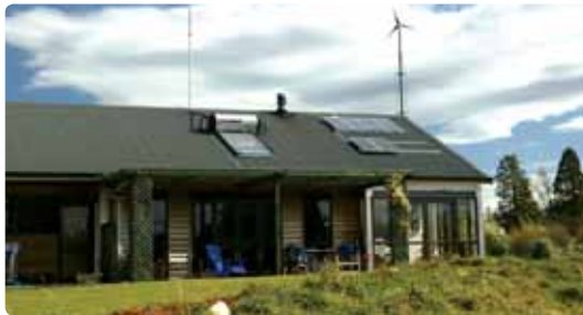
This photo shows a solar water heating system, solar photovoltaics, and micro wind turbine in a SAPS. Photo: EECA
