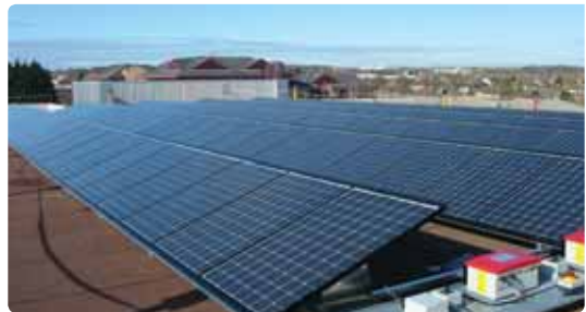
Frame mounted grid-connected PV system. Photo: www.solarcentury.com
