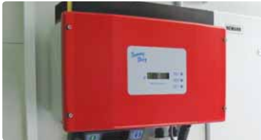
An inverter installation. Photo: SolarQuip Ltd.
