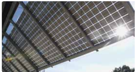
Photovoltaic 'glazing' can provide shade and electricity. Photo: www.solarcentury.com
