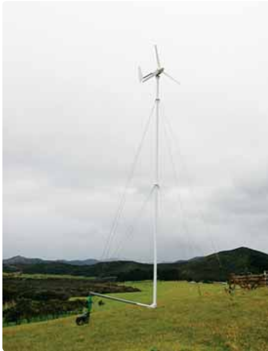
Pole mounted, with guy wires, three-bladed horizontal-axis micro wind turbine with a tilting mechanism. Photo: Gusto Energy Ltd.
