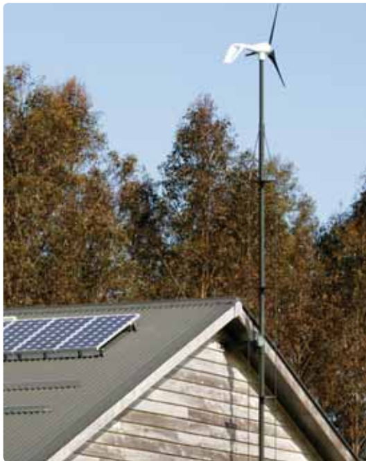
Micro wind turbine on a self-supporting tower next to a house. Photo: EECA
