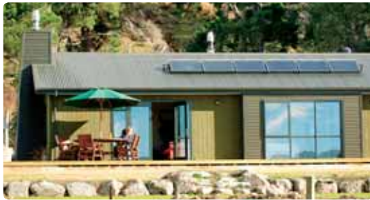
A solar water heating system installed with a stand alone power system. The house does not have a connection to the electricity network.
