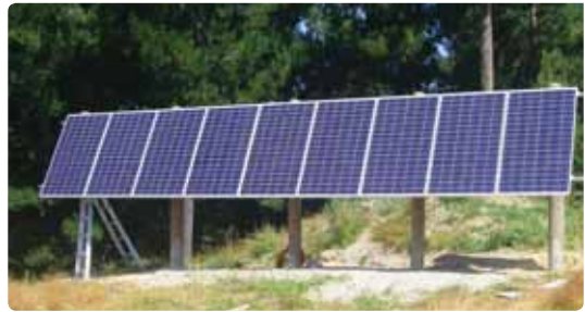
A ground mounted photovoltaic array. Photo: www.powersmartsolar.com
