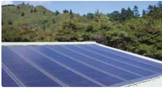
An example of photovoltaics with a flexible substrate. The sheets are rolled directly onto the roof. Photo: Alice Leney
