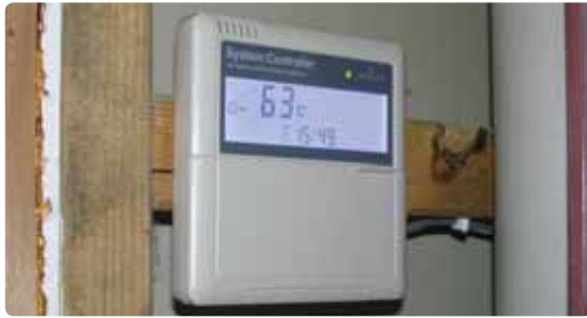
A typical controller for a solar water heating system.
