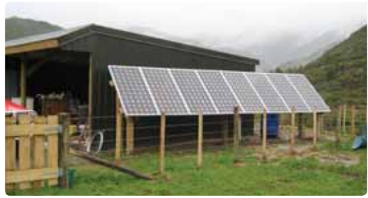
An example of a frame-mounted PV array on the ground. Photo: Ecogise
