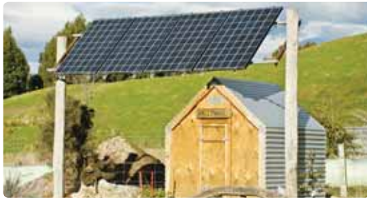
A ground mounted PV array in a SAPS. Photo: EECA
