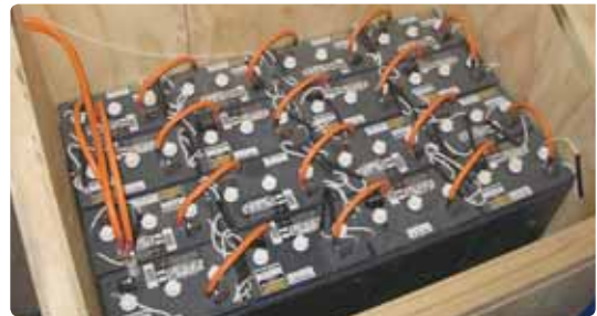
The batteries for this SAPS are well protected and secured in this box, preventing unauthorised access. Photo: SEANZ
