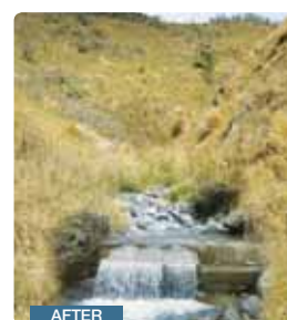
Simulation of the impact a micro (2-5kW) hydro scheme could have, looking upstream. A small weir is constructed to divert a portion of the stream into a penstock. Photos: Genkit Nelson Ltd.
