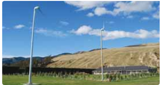
Two wind turbines on monopoles, in a grid-connected system near Christchurch. Photo: EECA
