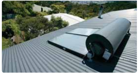
A residential thermosiphon solar water heating system.
