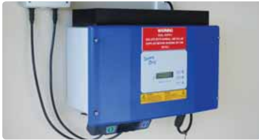
An inverter. Photo: www.powersmartsolar.com
