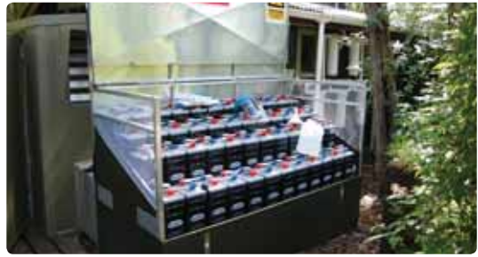
Another example of a battery bank on a SAPS. Photo: Genkit Nelson Ltd.
