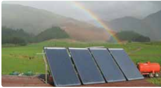
Frame-mounted solar water heating collector panels installed on a dairy shed.
