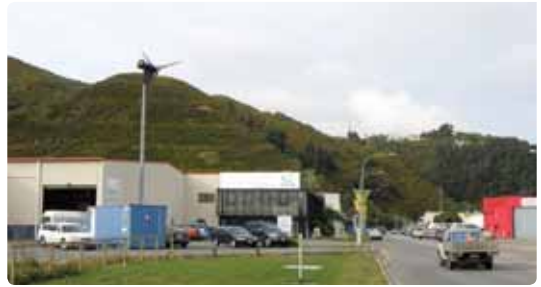
A three-bladed downwind turbine on a 15m high tubular pole. Photo: Proven Energy New Zealand
