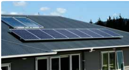
A PV array installed directly onto the roof. Photo: www.powersmartsolar.com
