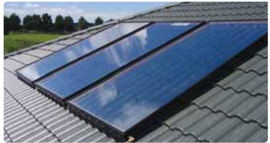
Frame-mounted flat plate collector panels.
