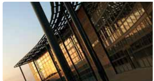
Photovoltaic 'solar louvres'. Photo: www.solarcentury.com
