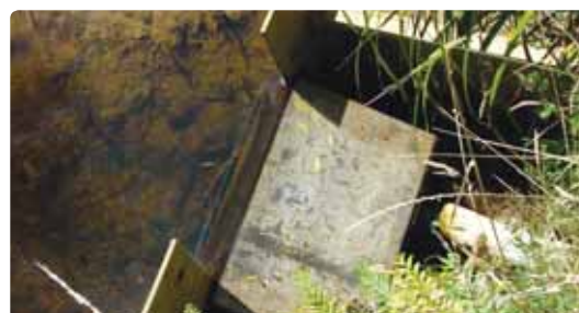
Another example of an intake structure. The stream flows over the metal screen, which prevents leaves or debris from entering the white plastic penstock. Photo: EcolInnovation
