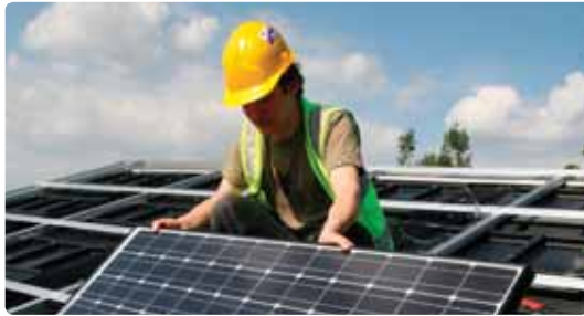
PV modules can replace conventional roof cladding. Photo: www.solarcentury.com
