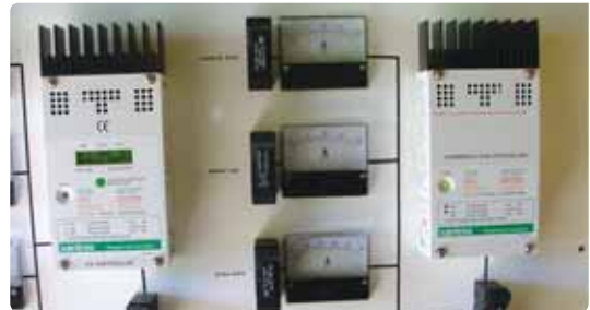
Examples of controllers for a PV array. Photo: EcolInnovation
