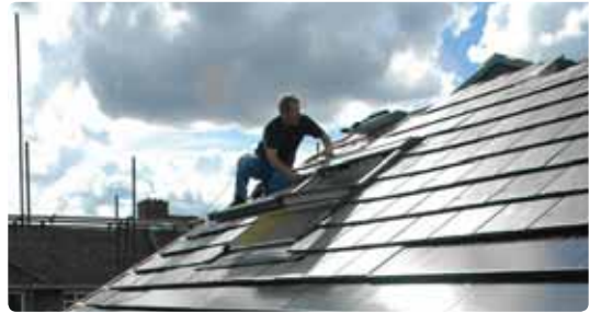
PV roof tiles. Photo: www.solarcentury.com
