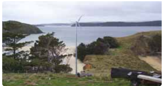
Self-supporting tubular tower mounted three-bladed horizontal-axis micro wind turbine. Photo: Elemental Energy
