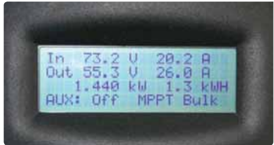
Example of a display unit on a grid-connected photovoltaic system. Photo: www.powersmartsolar.com
