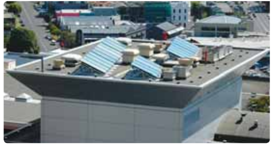
A commercial-scale solar water heating array installed on the Sky City building in Auckland.
