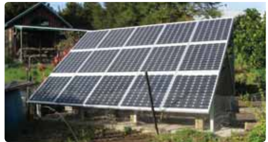
This photovoltaic array uses an inclined frame mounted on the ground. Photo: Genkit Nelson Ltd.
